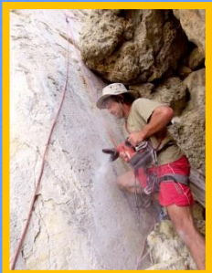
Xaqqa Valley Access Ladder
